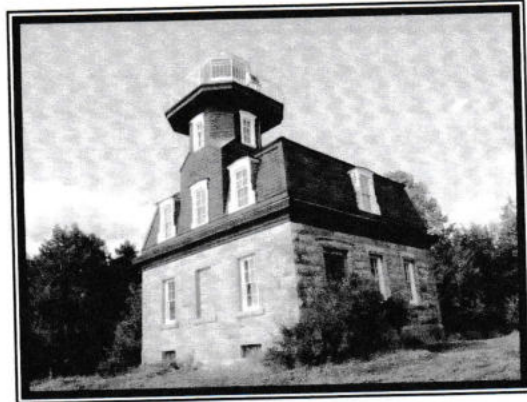
Summer - DEC Lighthouse Restoration
